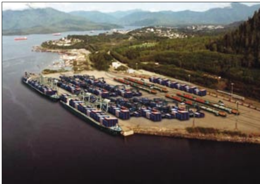
The future two-berth, 400,000-TEU container terminal at Prince Rupert Port, directly on the transcontinental mainline of the Canadian National Railway.
