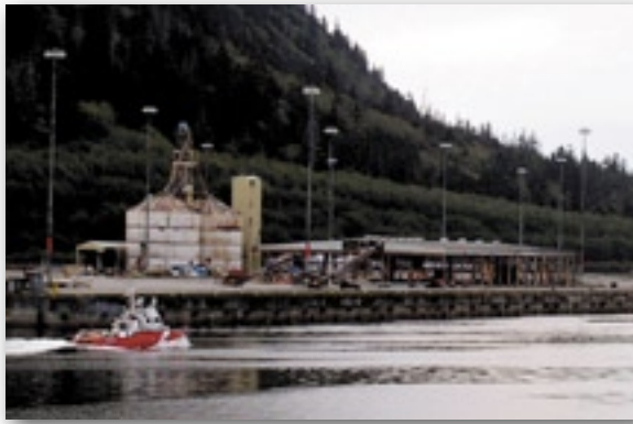
Fairview Terminal before demolition
