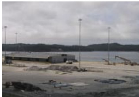
Fairview Terminal Demolition Progress
