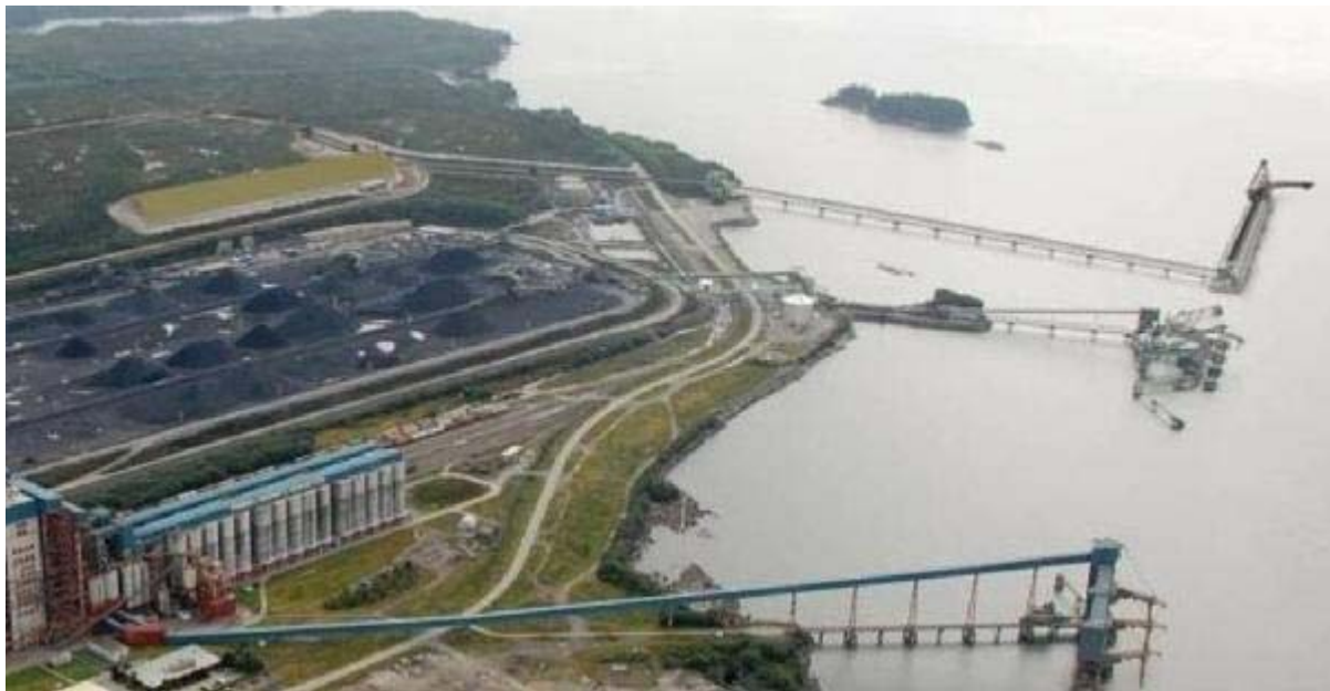
Artist Rendering of the Canpotex Potash Terminal (green building and berth above the coal terminal)
